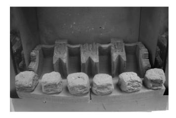
d) Fit four large coals behind the ceramic front rails as shown below in Fig. 6
