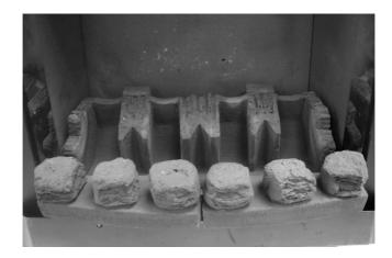
d) Fit four large coals behind the ceramic front rails as shown below in Fig. 19
